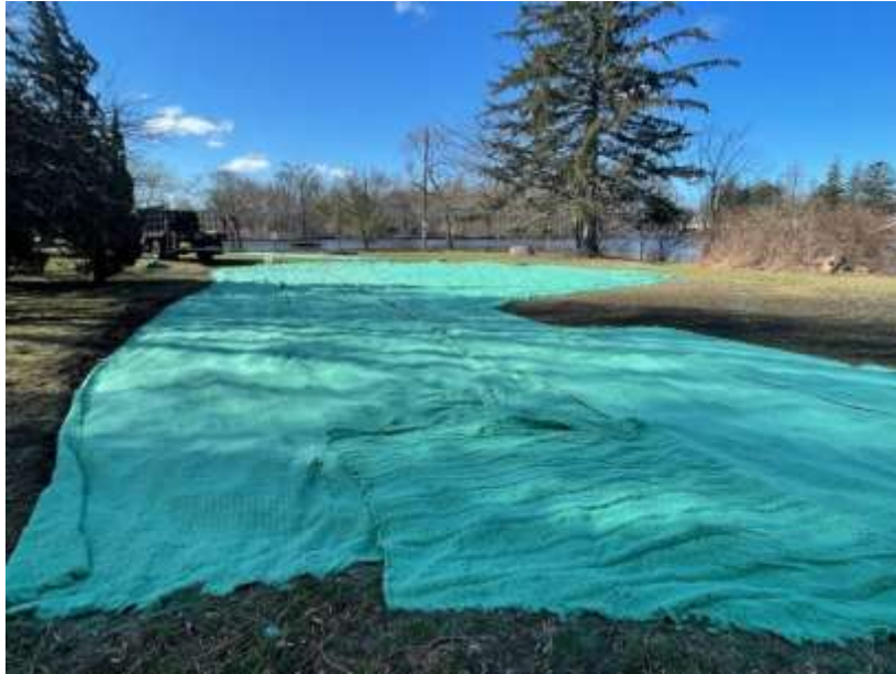
The "green cloth" installed
